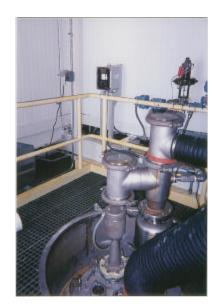
Ammonia Leak Warning – Sensidyne Gas Monitors Inventory Monitoring – Thermo Westronics Chart Recorders
