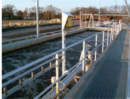
degradable organics in the wastewater. These microorganisms require air to survive and depend on the aeration system to provide the right amount of air necessary for them to thrive and consume the organics in the wastewater. Eventually, over a period of time,
